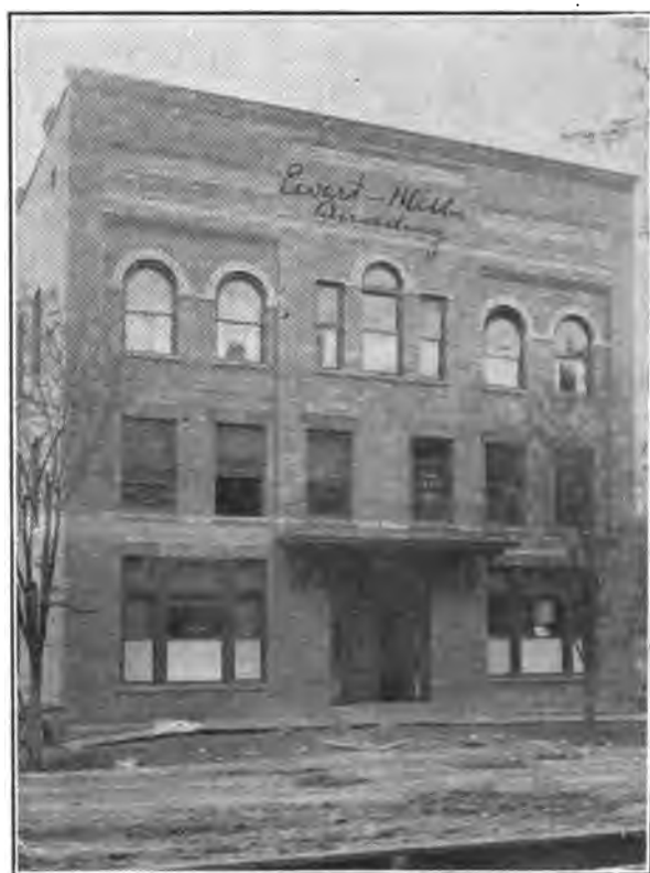
THE EWART-MILLER BUILDING. Erected in 1905.
